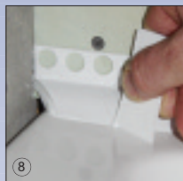
8 Remove excess Sealux-N off ledge if any
