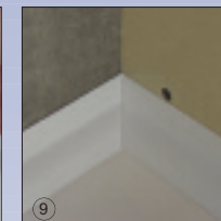
9 Ensure silicone fuses across corner joints.
