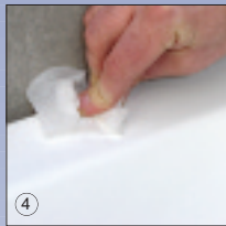
4 Clean ledge using Sealux alcohol/meths wipes
